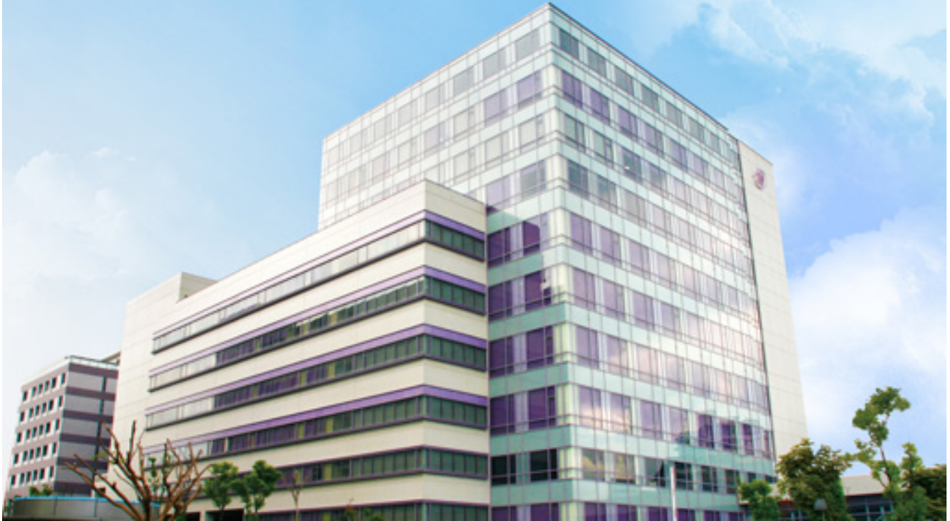
Portwell Engine (PE) Building
